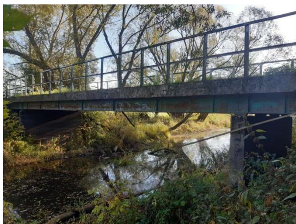
Fot. 97 Most Parking
